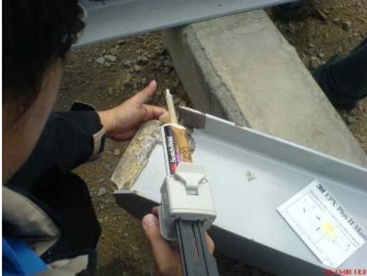
Figure 4: handheld 3M™ EPX™ Plus II applicator containing a duo-pak cartridge with attached static mix nozzle.
