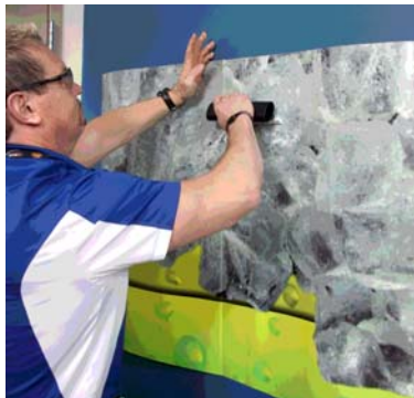
FIGURE 14 Squeegeeing Exposed Adhesive for Self Hinge
