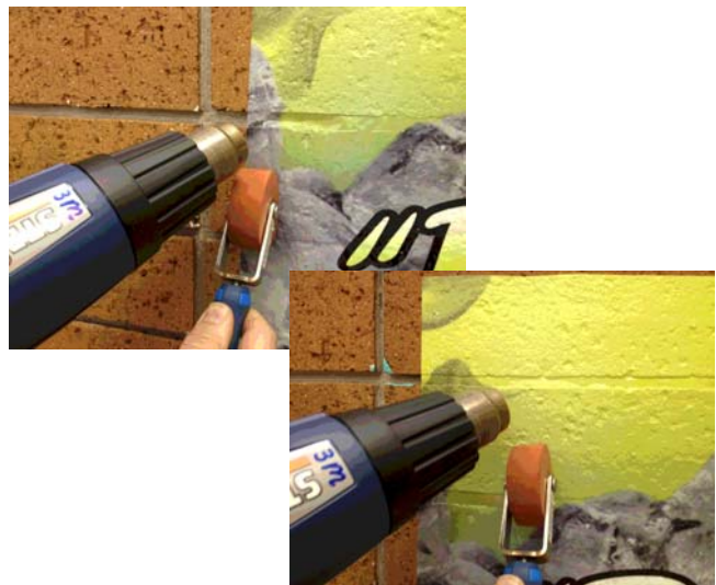
FIGURE 32 Use the TSA-3 Tool and Heat Gun to Touch Up Poorly Adhered Areas
