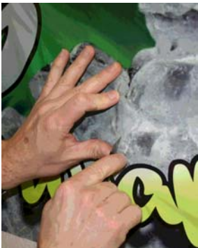
FIGURE 36 Cut Away Film a Little at a Time
