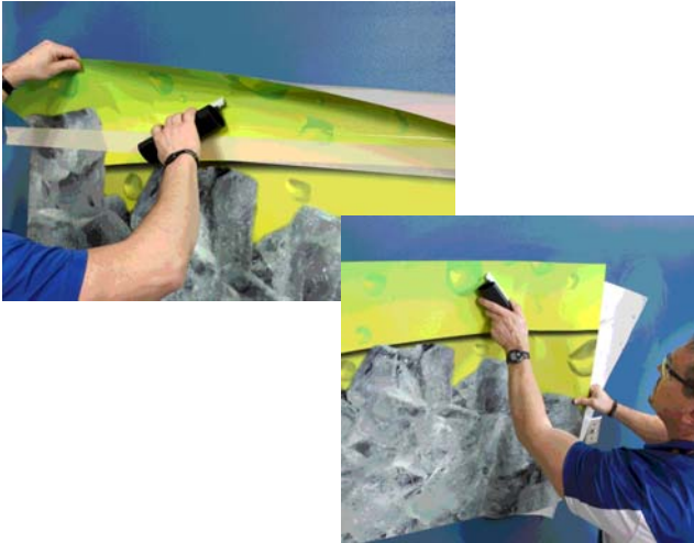
FIGURE 17 Keep Tension on the Unapplied Film
