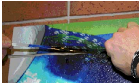
FIGURE 33 Cutting Film From Grout Lines
