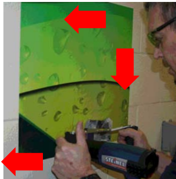
FIGURE 28 Lightly Set 3 Film Edges
